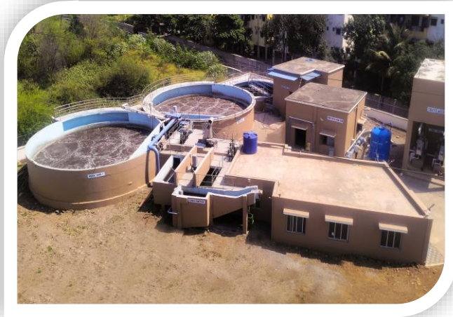
SEWAGE TREATMENT PLANT
